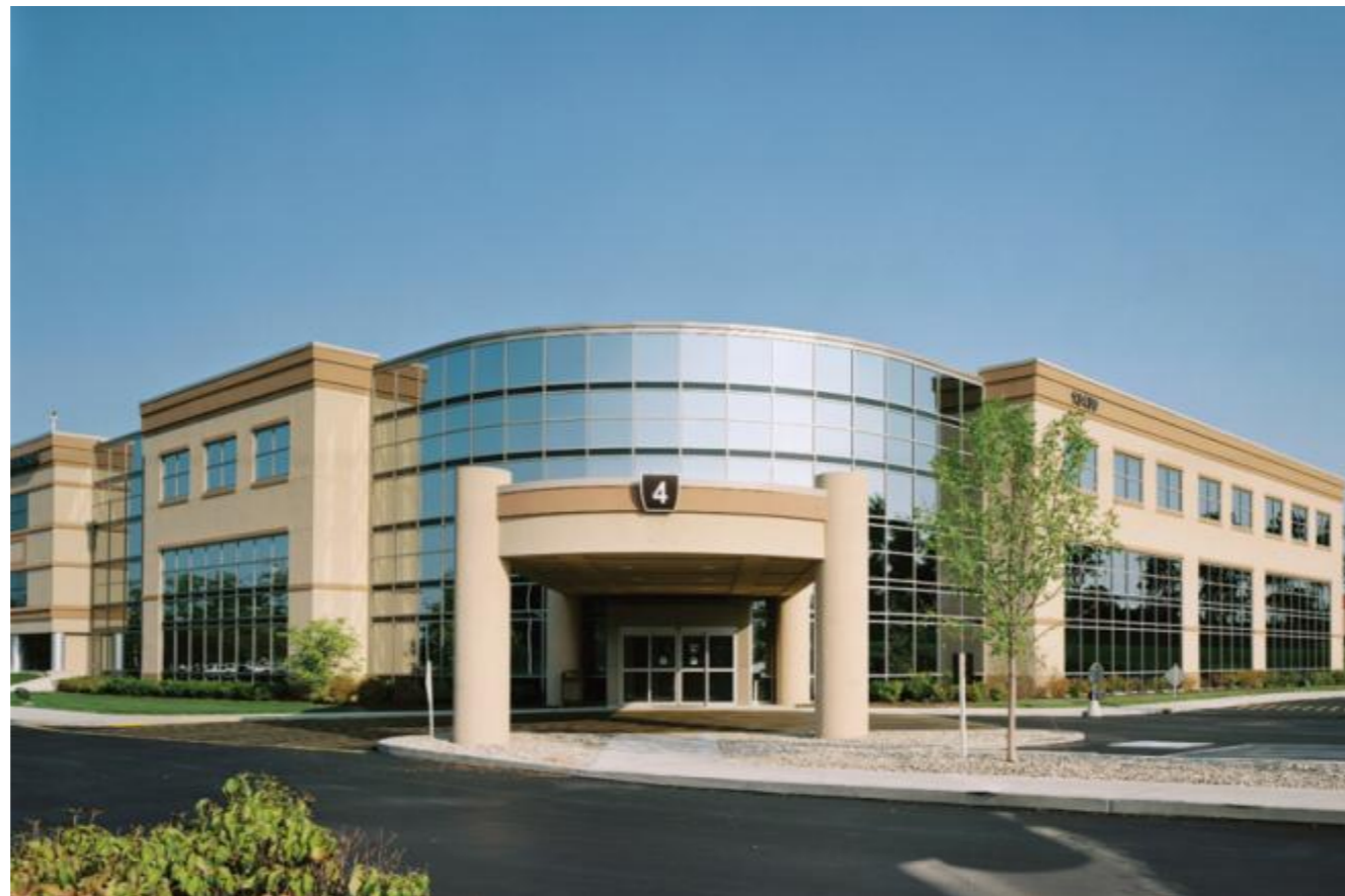
Professional Office Building - Carmel, Indiana
